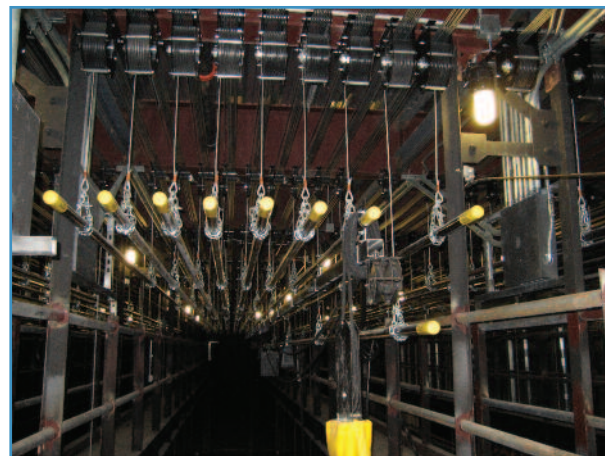
This is a modified gridiron with careful design and coordination of the catwalks to permit maximum fly space and some effects and spot lines in a 50'-high stage. Electrics and the orchestra shell fly in the space under the catwalks.
